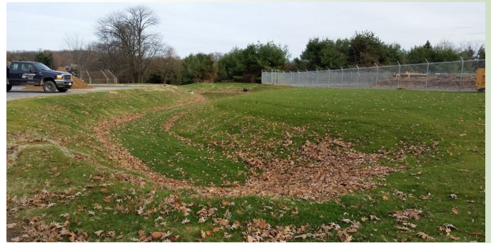
Rain garden BMP at the North Lebanon Township Yardwaste Recycling Facility
