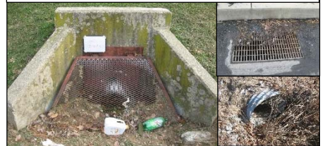
The below stormwater facilities require proper maintenance and removal of trash and debris.
