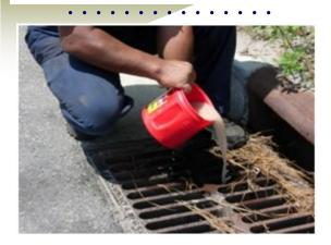
An illicit discharge is "any discharge to an MS4 (Municipal Separate Storm Sewer System) that is not composed entirely of stormwater..." Illicit discharges are considered "illicit" because MS4s are not designed to accept, process, or discharge such non-stormwater wastes.
